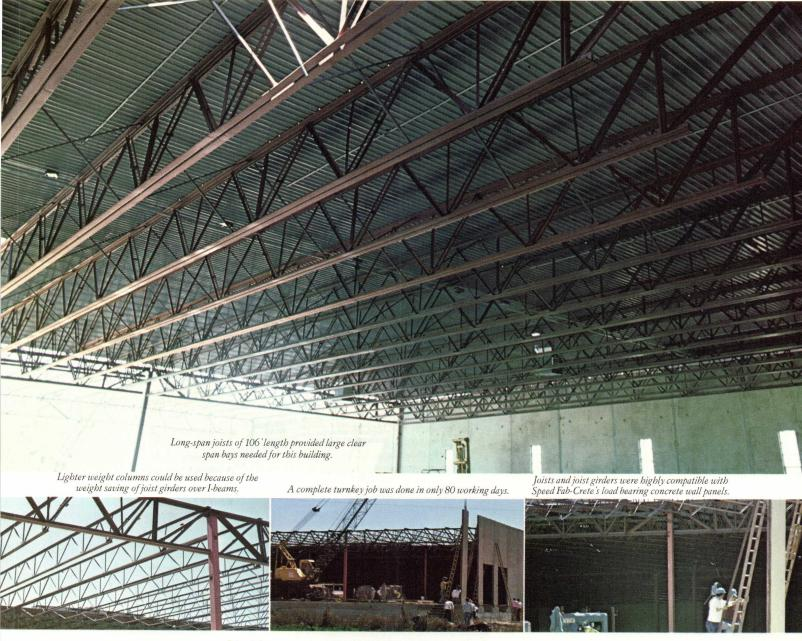
Joist girders were engineered and designed to meet the particular requirements of this job.
