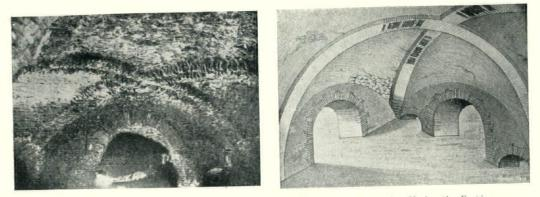
Two illustrations from Roman Architecture and Its Principles of Construction Under the Empire descriptive of ribbed cross-vaulting
